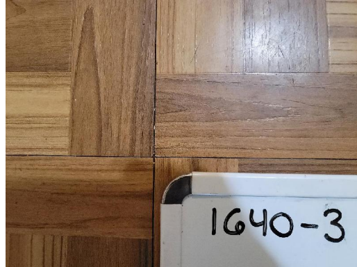
1640-3 12"x12" Floor Tile/Mastic Interior Kitchen (60 sq. ft.)
